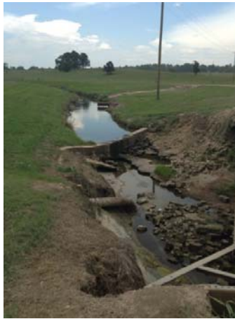
Figure 7 | Evidence of low sinuosity, active unstable streambanks, undercutting and streambed erosion/outcrop along the main stream and below a hydraulic structure in a tributary of the Red Bud – Catalpa Creek Watershed.
