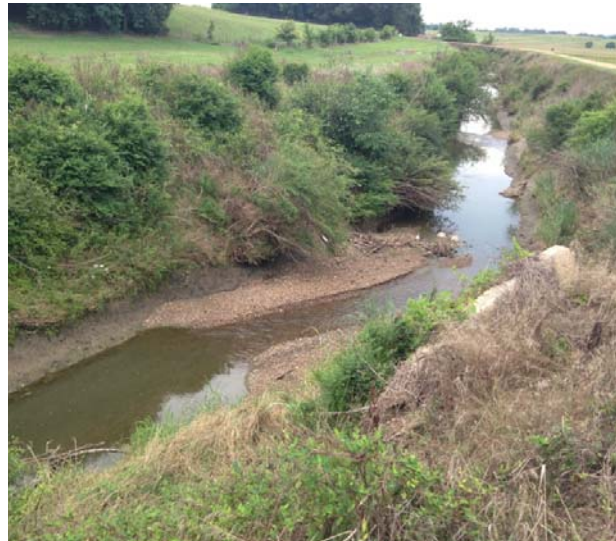
Figure 7 | Evidence of low sinuosity, active unstable streambanks, undercutting and streambed erosion/outcrop along the main stream and below a hydraulic structure in a tributary of the Red Bud – Catalpa Creek Watershed.
