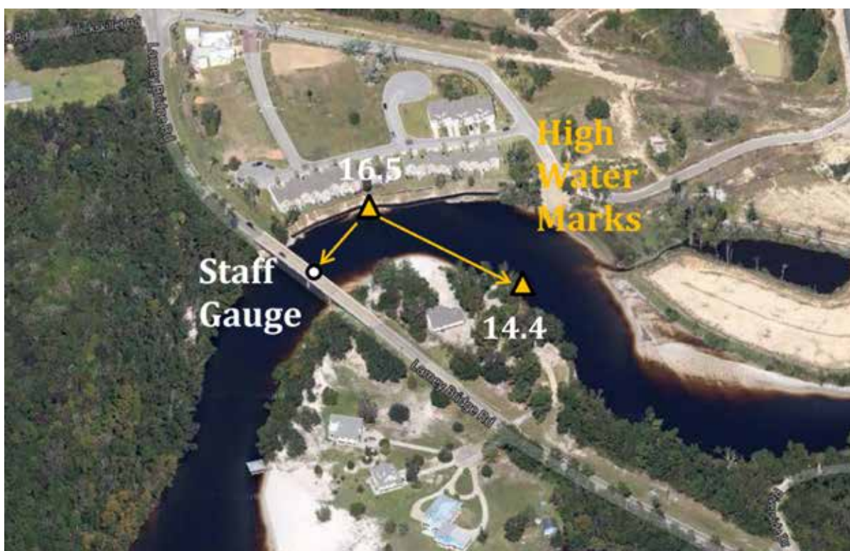
Figure 12. High water marks near the Tchoutacabouffa River at Lamey Bridge Rd (DIBM6).
