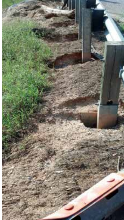
Figure 5. Guardrails on downstream side of the Silver Run Rd. bridge showing evidence of scouring.
